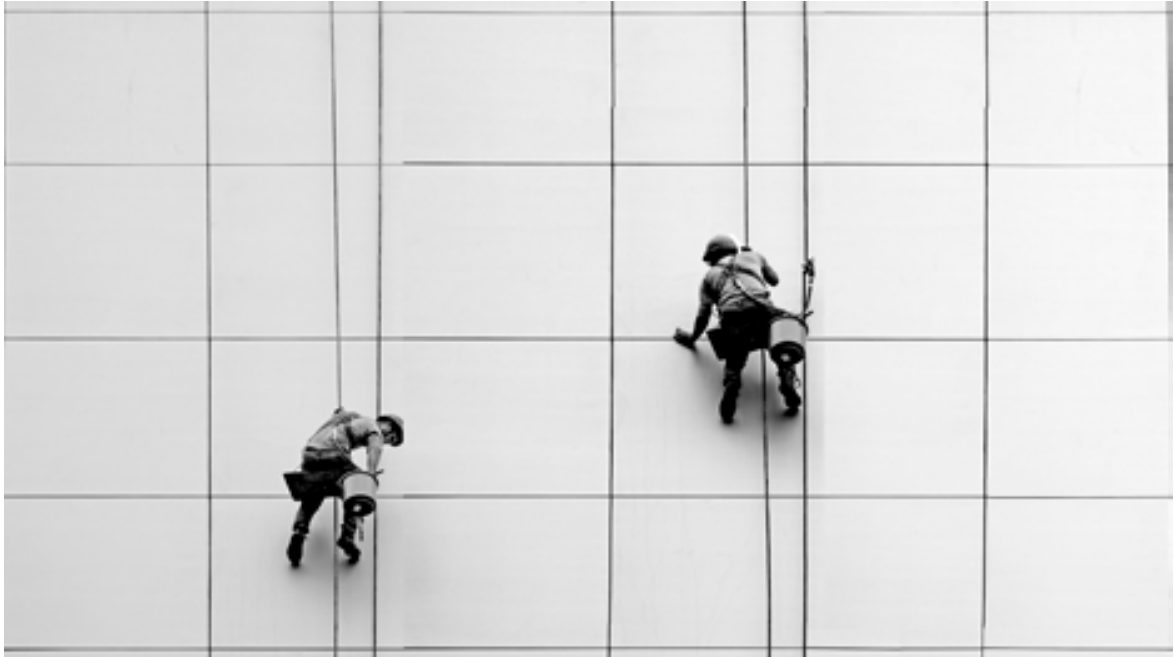
Paint renovation H.W. CHAN - Hong Kong
